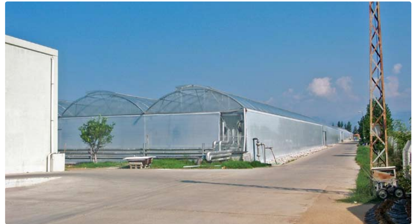
Arched Roof Greenhouse - Antalya, Turkey
